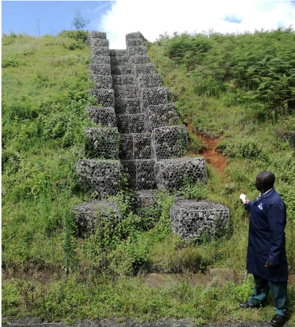
Plate 3. Emergency spillway
