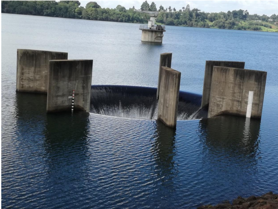
Plate 2. Main spillway with intake tower in the background
