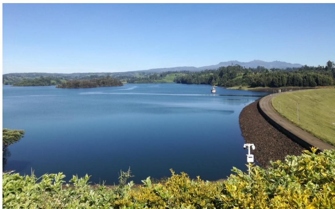
Plate 1. Thika Dam and reservoir
